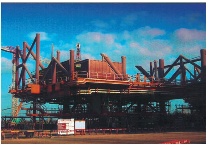
Work on the topsides at J Ray McDermott's Jebel Ali yard.
