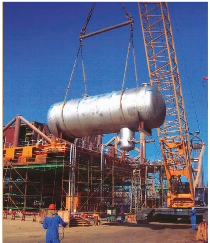
A knockout drum is lifted into position
