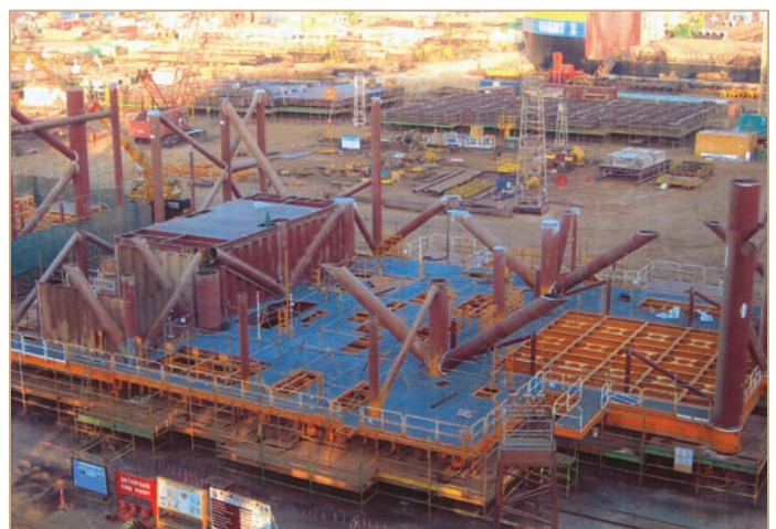
Work on the topsides at J Ray McDermott's Jebel Ali yard.
